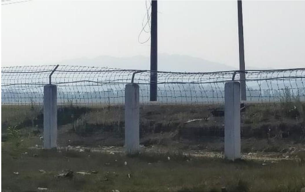
**Photo 29: Fencing for Boundary Protection**
